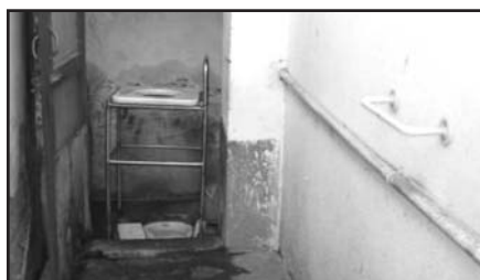
Toilet after modification
