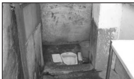
Toilet before modification
