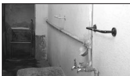
Hand rails nailed on the wall
